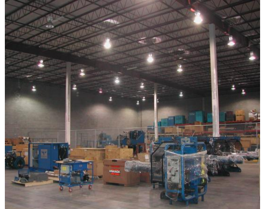
Figure 2: Conventional highbay fixtures are often used to provide illumination for large commercial facilities with ceiling heights of over twenty feet.
