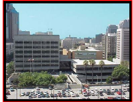
County of Sacramento Administration Building
