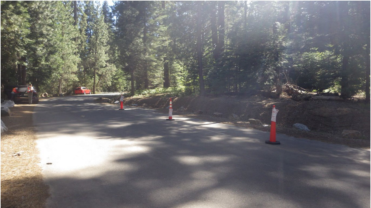
Figure E-13. North Union Valley Road during the peak season (6/10/22) with designated parking spots closed for construction and three vehicles parked on the side of the road.
