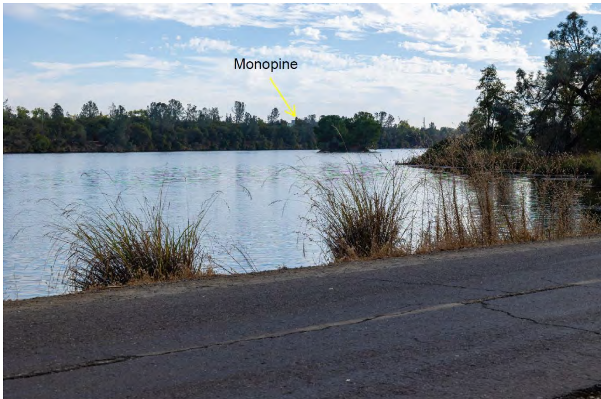
Figure 4c Viewpoint 4: View from the American River bike trail with the proposed monopole tower disclosed on the project site.
