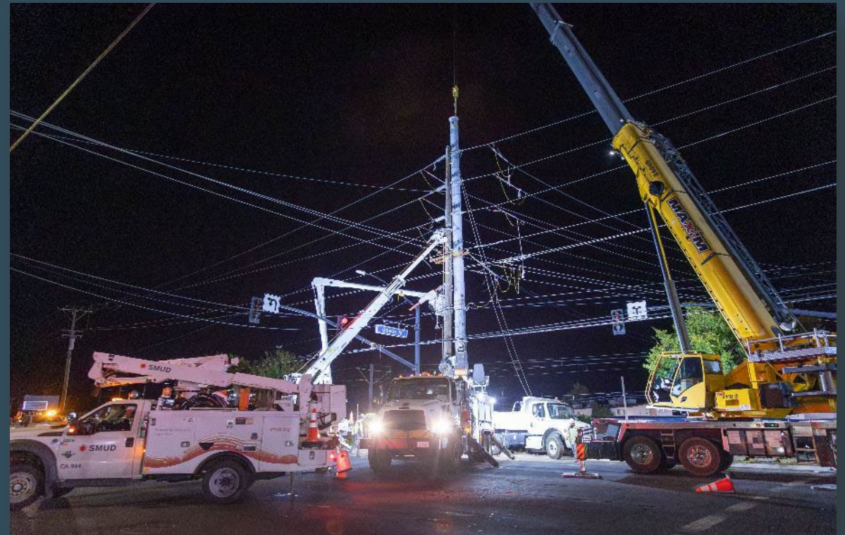
Line crew replacing 90 ft. steel pole – Folsom Blvd.
