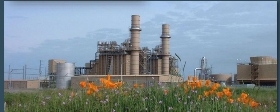
Cosumnes Power Plant
