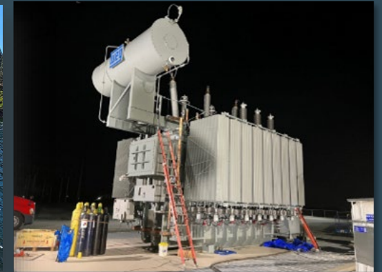
Transformer Replacements
