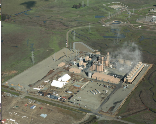
Cosumnes Power Plant
