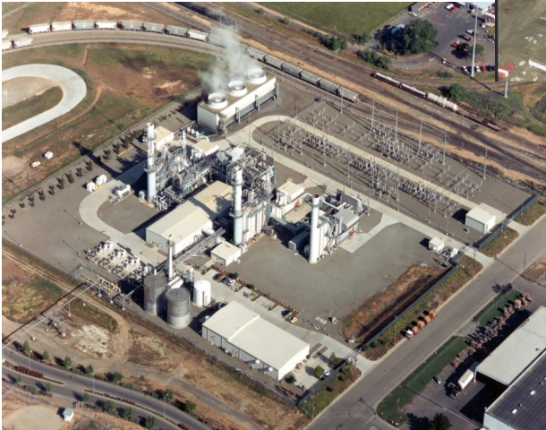
Procter & Gamble Power Plant
