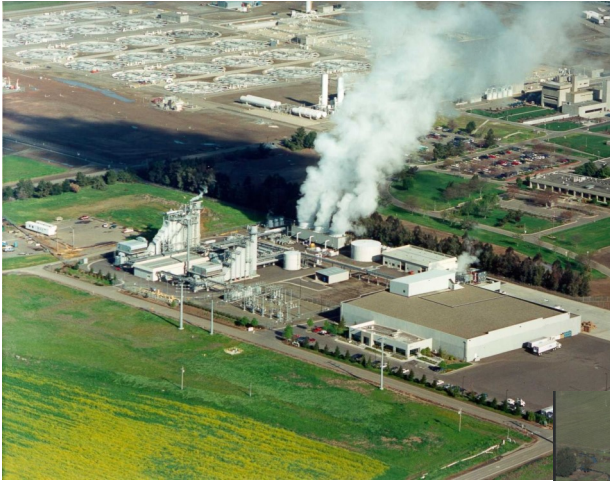
Carson Power Plant
