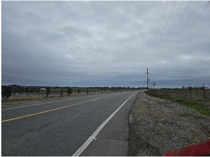
Photograph 3 Route of Transmission Line at Excelsior and Florin Roads
