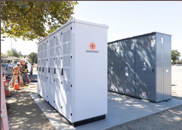
Construction underway at Sac. State
