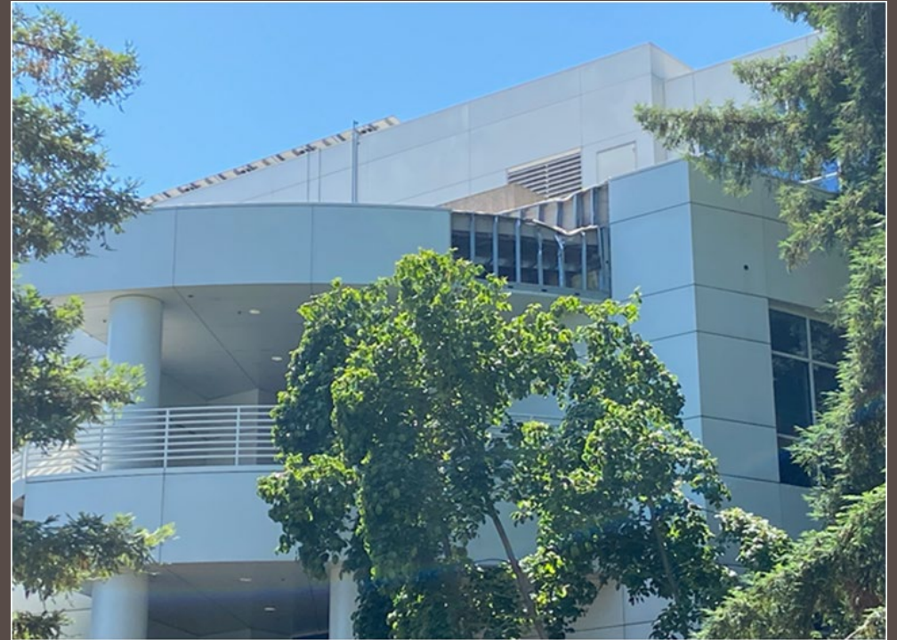
SMUD Customer Service Center Renovation
