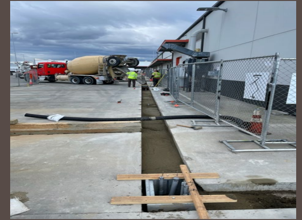
Site Work – EV Charging
