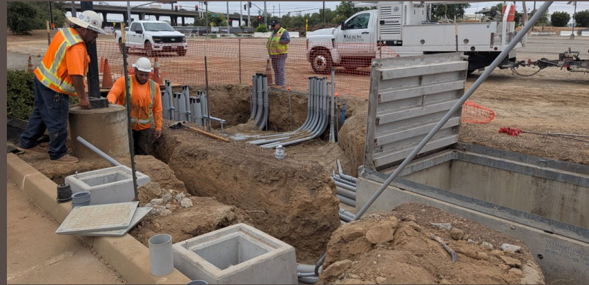
FAST construction of 6x public DC Fast chargers at CSUS
