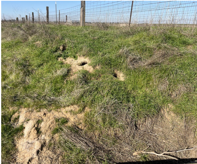
Photograph 1. Burrow complexes in the southern portion of the project site. AECOM 01.15.2025
