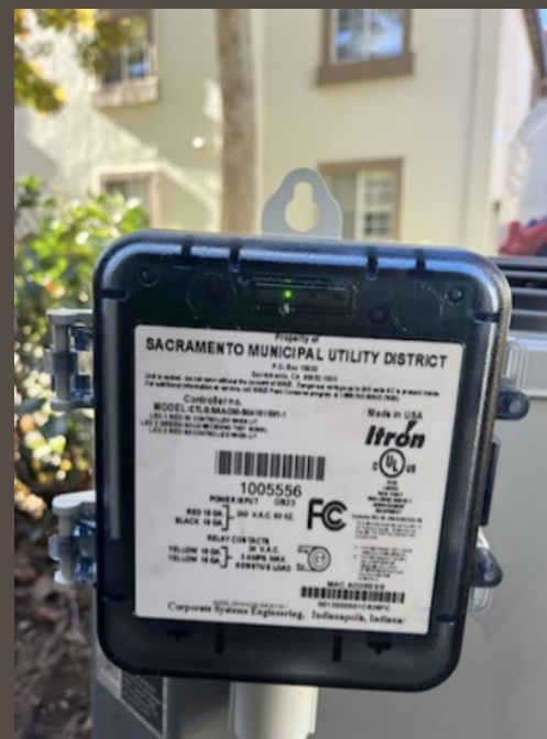
Peak Conserve switch installation
