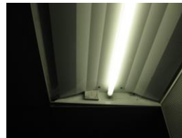
Figure 5: The original lighting system had been de-lamped as part of a previous energy efficiency project
