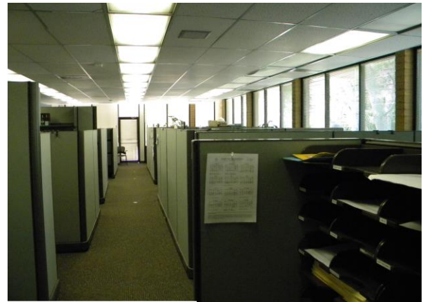
Figure 5: The original lighting system had been de-lamped as part of a previous energy efficiency project
