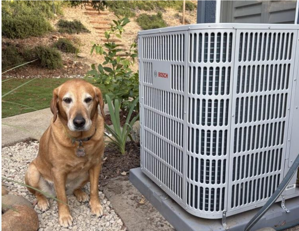
Advanced Home Solutions: Happy Customer with a new heat pump HVAC
