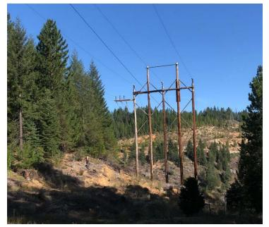
60kV wood pole design with 4kV attachment
