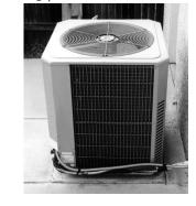
equipment will operate in short run times or cycles, not allowing the unit to reach efficient operation or deliver even temperatures throughout your home. A right-sized unit will provide more comfort and cost less to operate than an oversized system. Title 24 energy code and SMUD program require sizing by an engineered load calculation method.
