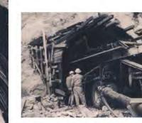
Workers check the progress of a drilling rig during the first construction stages of the Jaybird Tunnel in September 1958. The drilling lasted approximately 2 years as the tunnel grew to nearly 4 miles.
