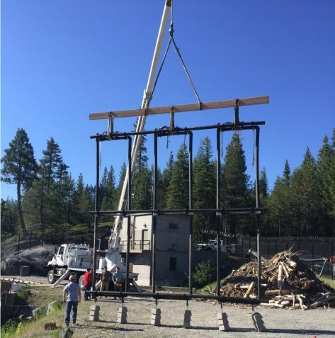
Figure 4. Vertical antenna group prepared for deployment at Robbs Peak Forebay trash rack.
