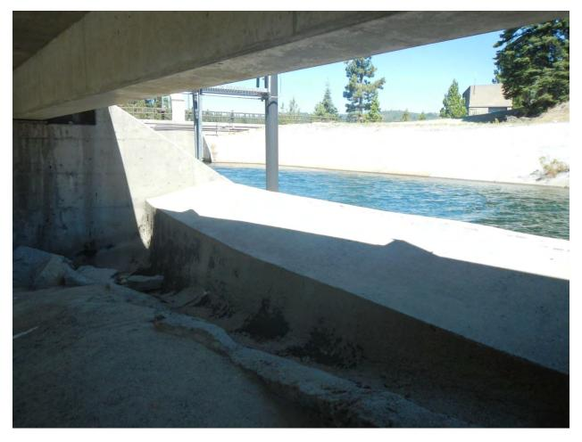
Photo 3. Looking north from below the bridge at the spillway outlet. Note the concrete lining at the outlet.
