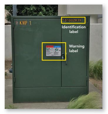
Actual locations of labels may differ on each box. All labels must remain visible after wrap is installed.
