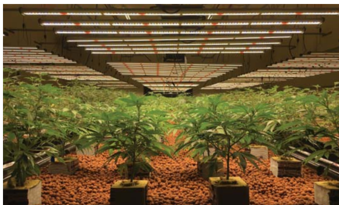
LED fixtures installed in room 2.
