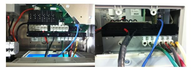
Figure 4-5. Inverter with power and communication connections
