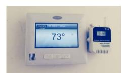
Figure 8 Wireless Temperature Logger Mounted Next to Carrier Thermostat (PCT).
