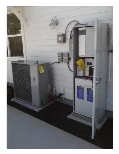
Figure 3 Sunverge SIS unit (Door Open) on the Right and Air Conditioning Unit on the Left.
