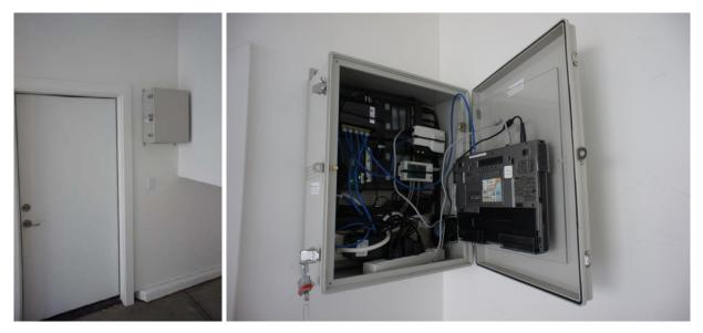
Figure 6 Box Mounted in Garage Containing Power Meters, Loggers and Laptop for Remote Data Collection.
