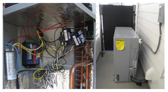
Figure 7 Air Conditioning Power Meter (inside) and Wireless Pulse Logger (outside).
