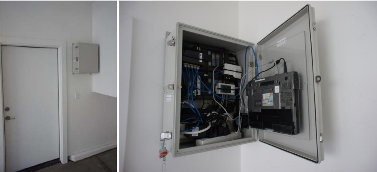
*Figure 6 Box Mounted in Garage Containing Power Meters, Loggers and Laptop for Remote Data Collection.*
