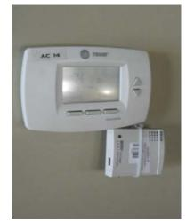
Hobo temperature logger attached to thermostat.
