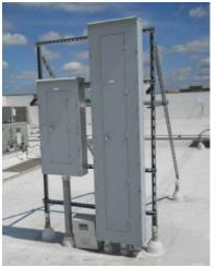
Power recorder mounted next to electrical panel on roof.
