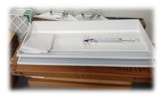
Figure 10: LED troffer disassembly to install wireless chip.
