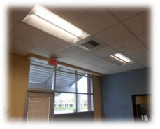
Figure 19: New LED lighting fixtures
