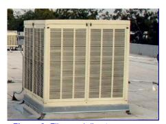
**Figure 2:** Fiber-pad direct evaporative cooler with aspen pads
