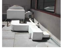
**Figure 7:** A poorly installed indirect-direct evaporative cooling system. The ductwork is far too restrictive to deliver the airflow needed to meet the cooling requirements of this classroom.<sup>6</sup>
