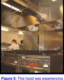
**Figure 5:** This hood was experiencing capture problems. CulinAire (the contractor) recommended installing a stainless steel back panel to help alleviate this problem.
