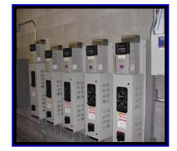
Figure 11: VFDs used to control the four of the exhaust fans and the make-up air handler fan.
