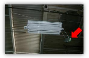
Figure 1-1: Steel plates installed below the sensor
