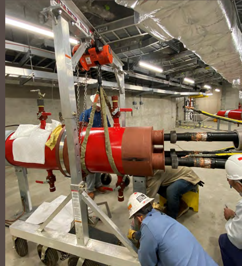
Transition Joint Line 1 Fault in Basement of Station G
