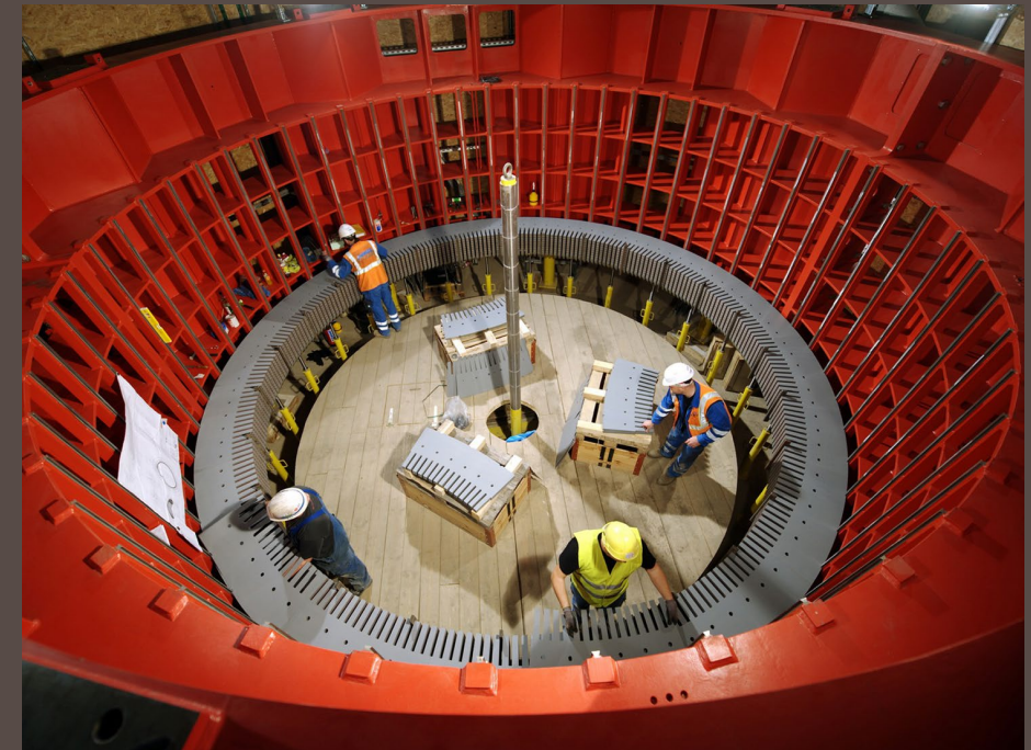
Piling the Stator Core
