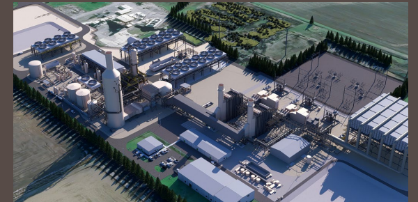
Sutter decarbonization project
