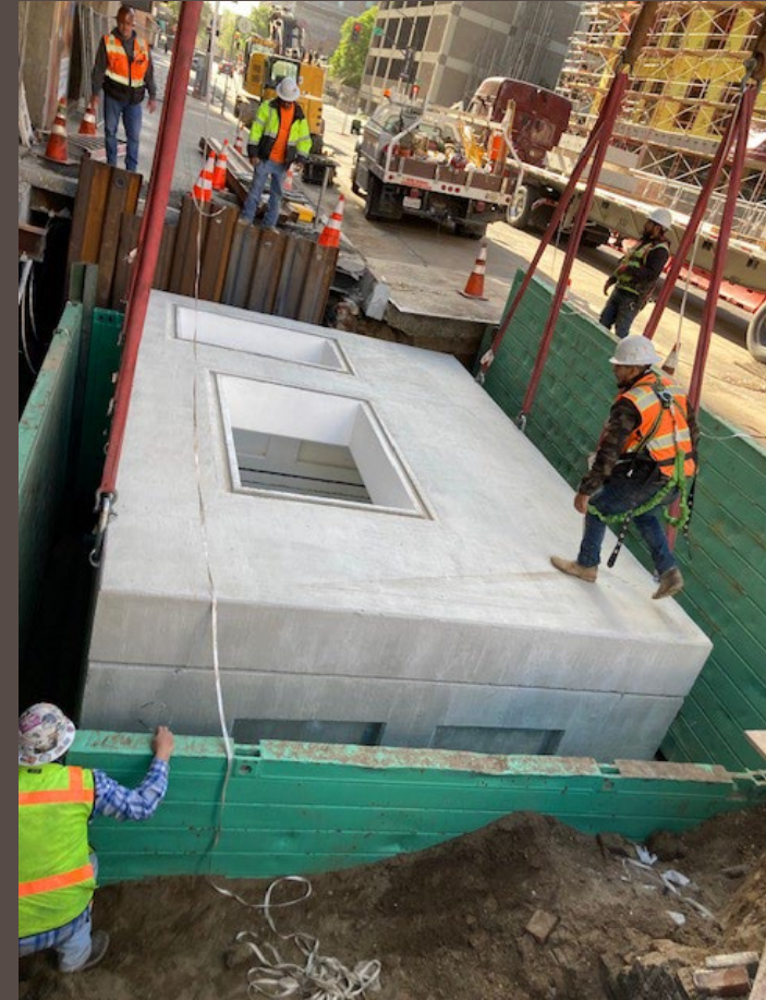
Splice Box for 21kV Underground Circuits
