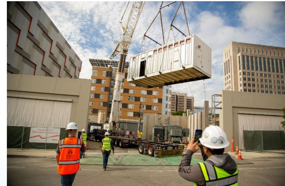
Switchgear building installation at Station G
