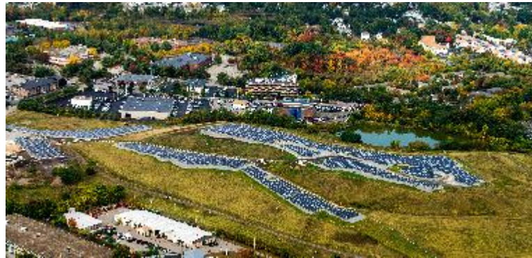
Grid Scale Energy Storage
