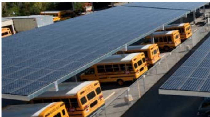
Solar+ES+EV Charging Microgrid
