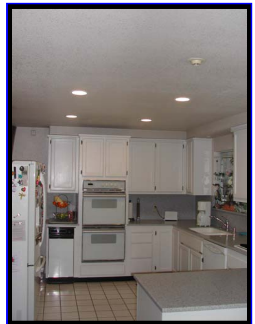
Figure 7: Customers who replaced surface-mounted, wooden, fluorescent light boxes with the LR6 experienced dramatic improvements in lighting quality as well as significant energy savings.
