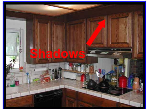
Figure 6: Most customers who replaced 4 ft. fluorescent fixtures had old-fashioned, surface-mounted, wooden light boxes. These systems tend to create shadows and make the room feel much smaller.
