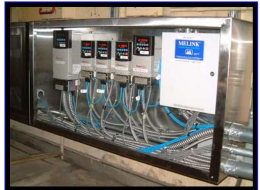
Figure 6: The VFDs and I/O processors had to be installed in a cramped attic mechanical room. This made installation a challenge.
