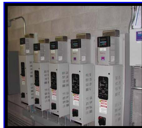
Figure 11: VFDs used to control the four of the exhaust fans and the make-up air handler fan.
