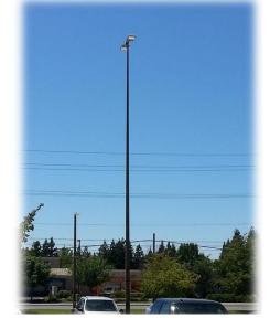
**Figure 1:** The new LED fixtures at Tri Tool Inc. were mounted at 50ft. above the ground, which at this time, was considered to be a challenging application for LED technology.
