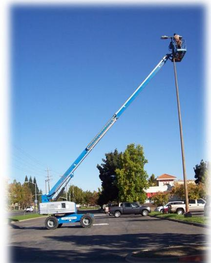
**Figure 6:** when the LEP fixtures failed prematurely, they were replaced with high output LED fixtures
