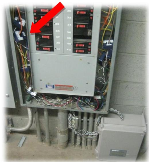
**Figure 9:** Split-core transducers were placed in the electrical breaker panel to measure the lighting system energy consumption.
