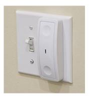
Figure 21: Since some of the residents wanted physical switches to control the lights the project team included several wireless switches like this one shown above.
