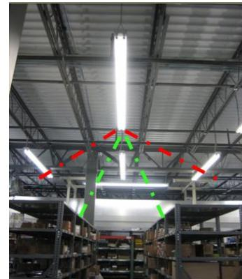
Figure 4: Finding a motion sensor with the right coverage patterns and minimum delay settings was a real challenge. Photo credit: SMUD
