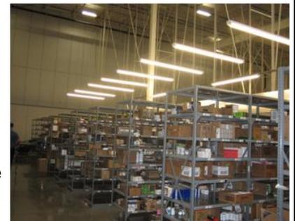
Figure 1: The original lighting system included hundreds of fluorescent fixtures. Photo credit: SMUD
