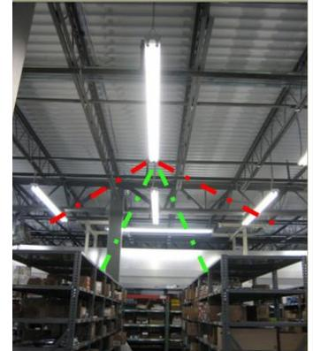
Figure 4: Finding a motion sensor with the right coverage patterns and minimum delay settings was a real challenge. Photo credit: SMUD
