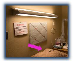
**Figure 18:** The push button switches for the LED overhead bed lights were too similar to the call light buttons.
