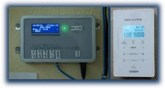
**Figure 15:** The controls for the LED cove lights (left) were much too complicated. The controls for the rest of the lighting were more intuitive yet lacked clear instructions.
