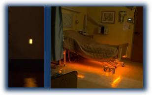
Figure 4: Amber LED rope lights and wall-mounted, amber LED nightlights.
