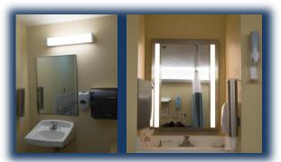
**Figure 5:** The original vanity lights produced a lot of glare (left side). The Project Team replaced these fixtures with dimmable, illuminated LED mirrors (shown on right).
