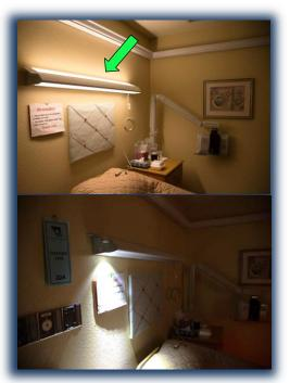
Figure 2: Direct-indirect, dimmable LED headboard fixtures provided light over the beds. These fixtures include a small LED spotlight to enable caretakers to read prescription labels and charts at night without turning on the main lights.
