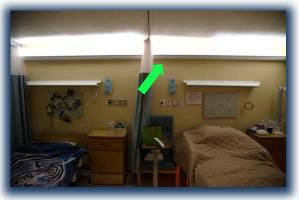
**Figure 3:** Tunable-white LED cove lights were installed in plastic gutters to shield residents from potential glare.
