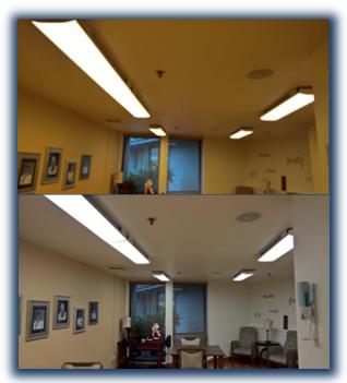
**Figure 9:** The family visitation room is illuminated by LED fixtures similar to the ones used in the hallways.
