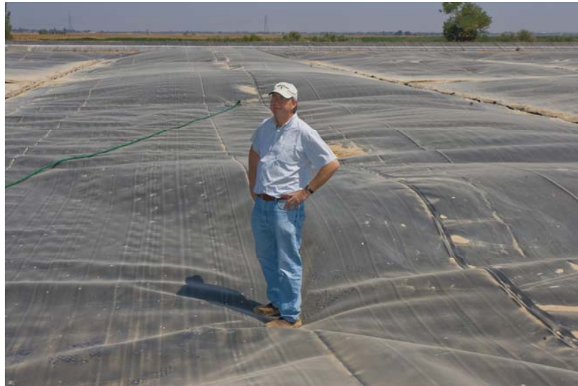
Suggested photo caption: This two-acre covered lagoon captures methane gas from cow manure that is then used to make electricity.
