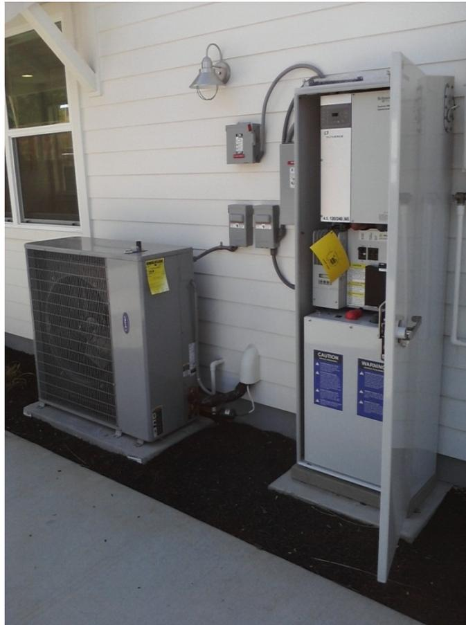
*Figure 3 Sunverge SIS unit (Door Open) on the Right and Air Conditioning Unit on the Left.*
